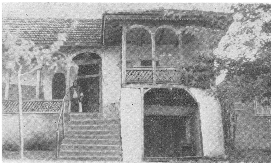
Fig. 13. — House with look-out tower built on a tall cellar's entrance (beginning of XX th century).
