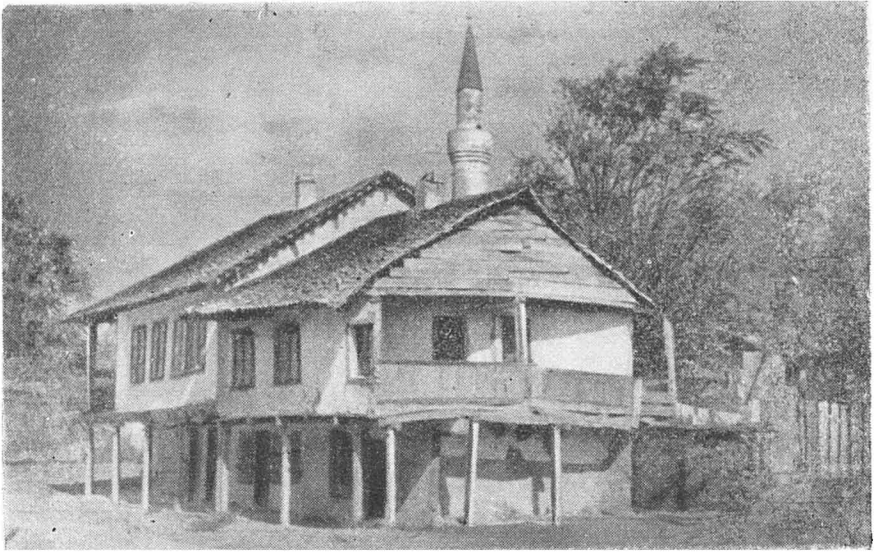
Fig. 19. — Storeyed-house built in console (beginning of XX th century).
