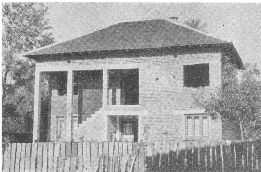
Fig. 23. — House in the building process.
