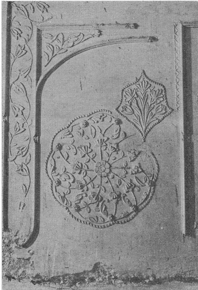
Fig. 10. — Decorative panel with restored stucco work. The Brancovan palace of Potlogi.
