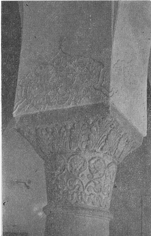
Fig. 9. — Detail of column with stucco work decoration. Princely house of Hurez.
