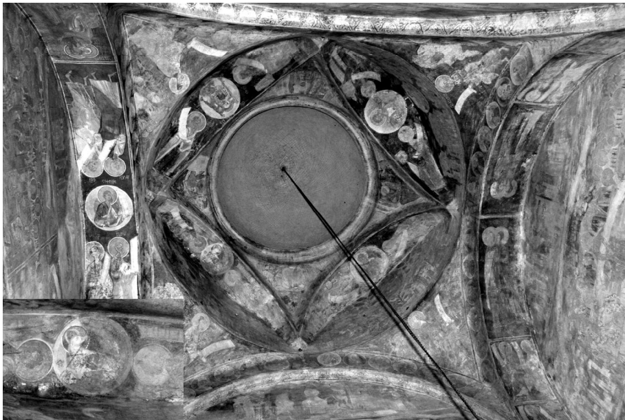
7. Dobrovaț, dome of the narthex; the Lamb is depicted on the north-western oblong arch – detail shown in vignette on the lower left corner (photo: V. Bedros).
