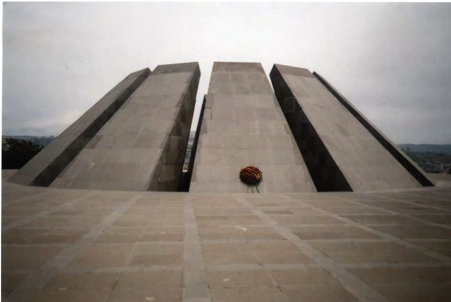
Fig. 15. The enormous hearth of the Genocide in Yerevan. View of the exterior and laying a wreath.
