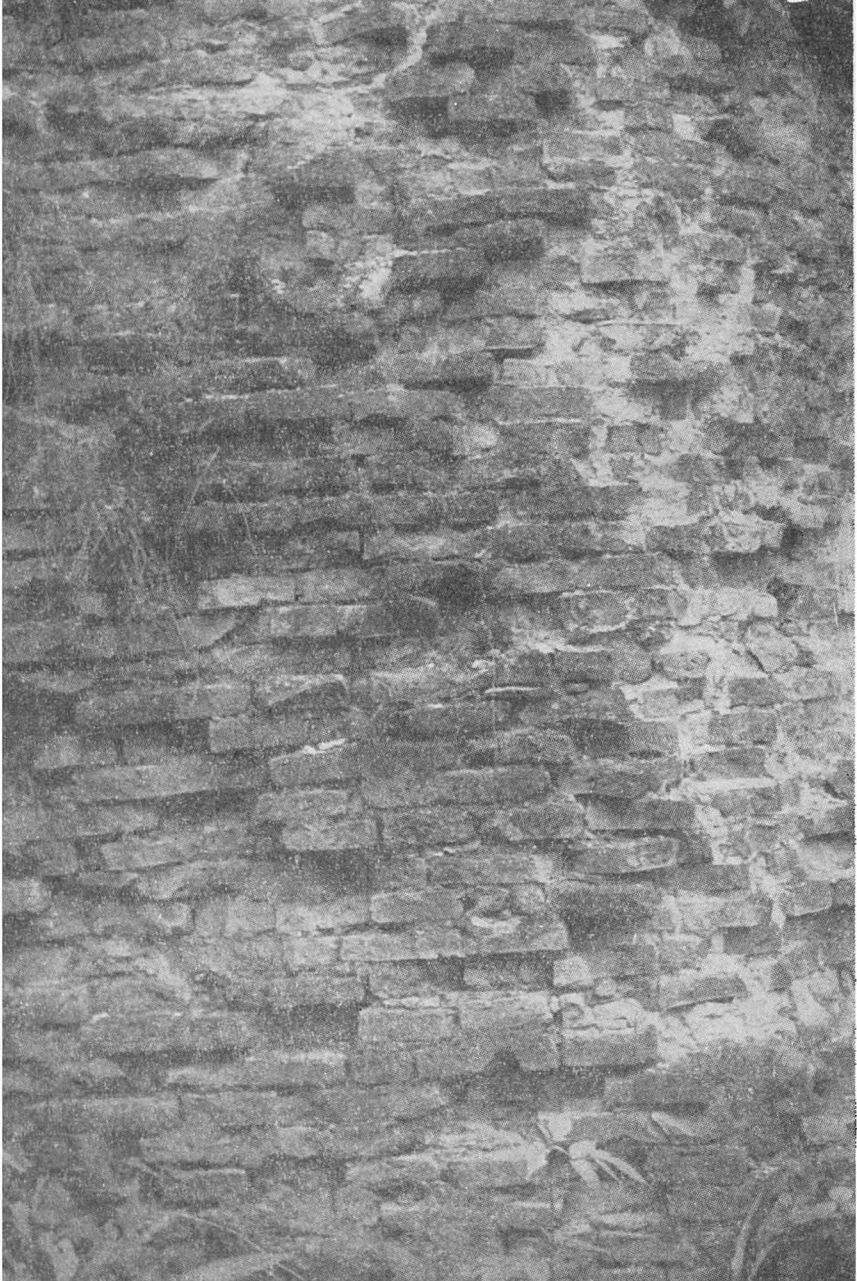
Fig. 2. — Castle of Kupinik, structure of masonry.
